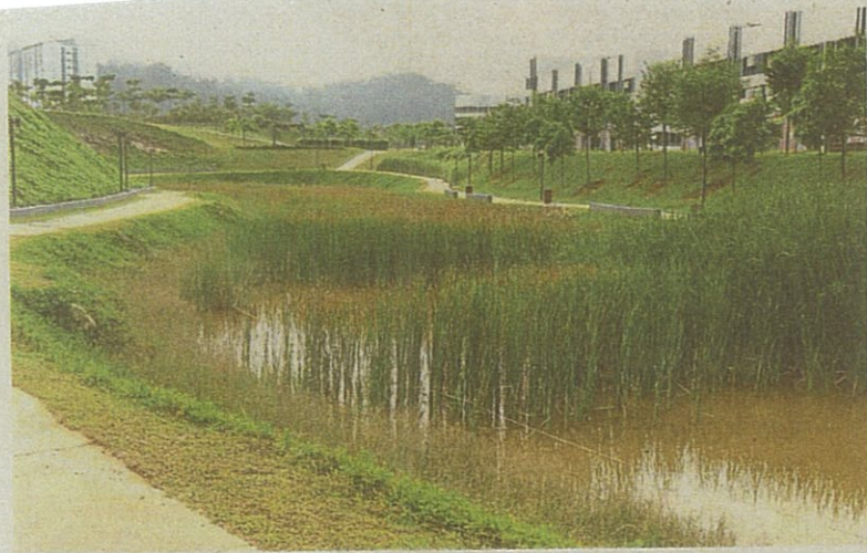
In areas like Setia Alam in Shah Alam, earth swale drains create surface channels to direct and slow down the movement of water, allowing it to be absorbed by the soil.
