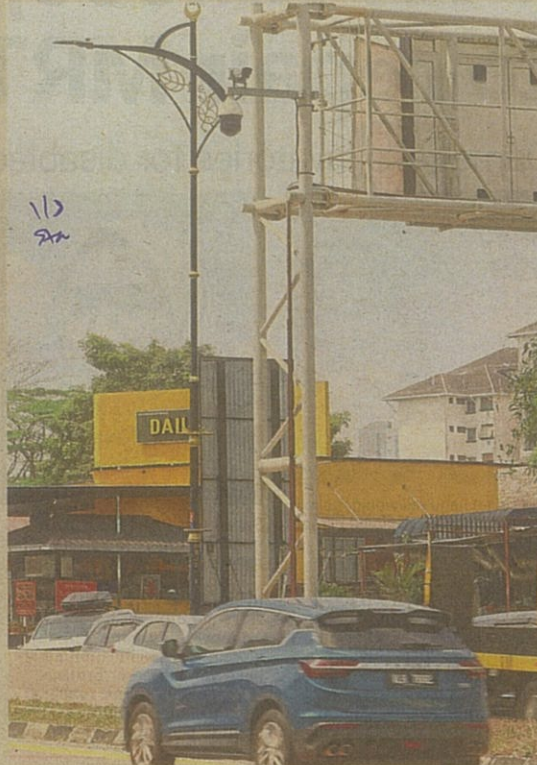
The smart camera system helps MJB and police monitor security and traffic flow within Johor Baru city.
