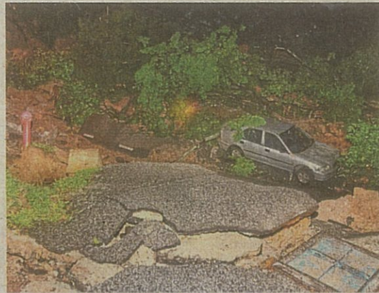
Nine terrace houses and four cars were affected in the landslide that occurred along Jalan Wawasan 3/9 in December last year. — Filepic
