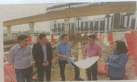
Ng (centre) discussing with the contractor on mitigation works done along Jalan Merbah 1 in Bandar Puchong Jaya. With them are Chong (second left) and Lee (right). — YAP CHEE HONG/The Star
