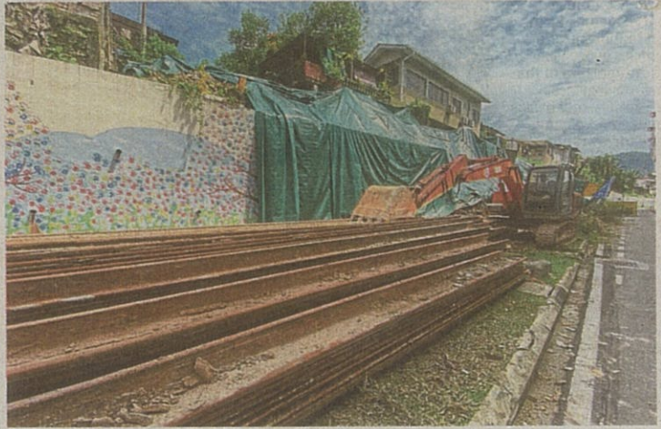
Dozens of sheet piles at the landslide site will be installed this week.
