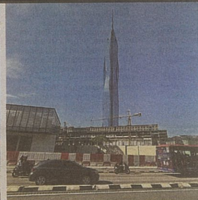
Menara Merdeka 118 towers behind the abandoned Plaza Rakyat project.
