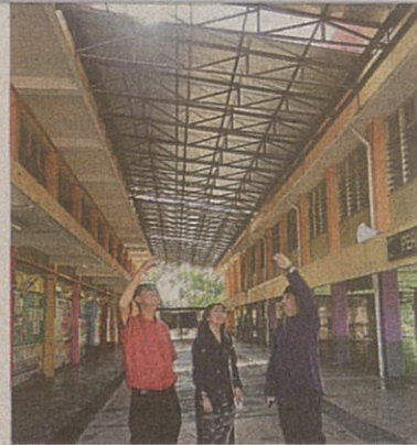
(From left) Ong, Lim and Wan Huzaini checking out the new skylight roof at SK Kampung Tunku. — LOW BOON TAT/The Star
