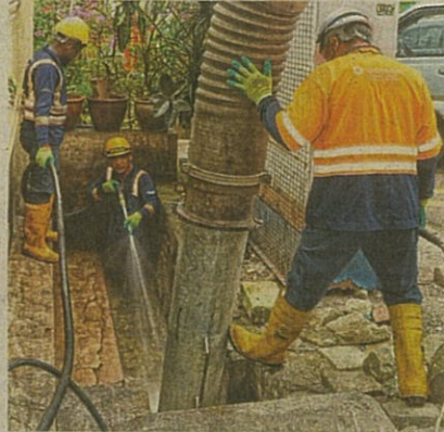
Alam Flora workers using a vacuum truck and water jet to clear a badly clogged drain in Kampung Baru, Kuala Lumpur. — Filepic
