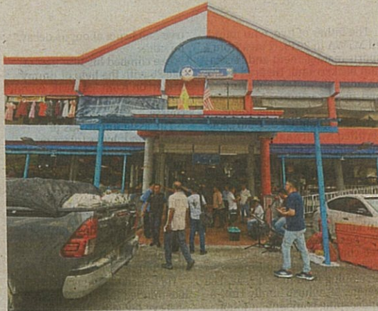
The market's facade has been painted as part of the upgrading works. — LOW LAY PHON/The Star
