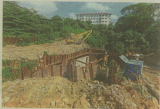
This Bandar Sri Damansara culvert project's contractor has been tasked to repair a slope nearby. — Filepic
