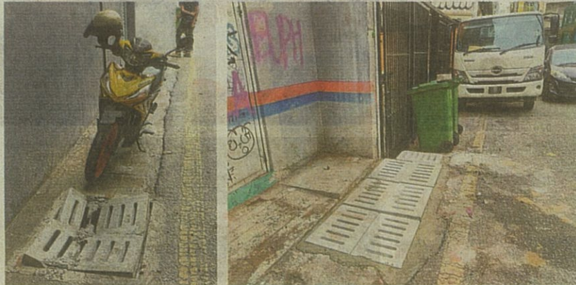
Drain covers before and after they were repaired in the back lanes of Jalan Alor in Bukit Bintang, Kuala Lumpur.
