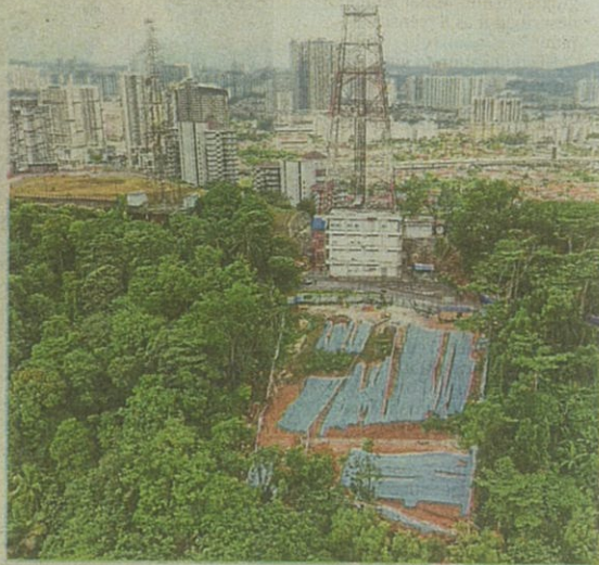
One of the Bukit Gasing bungalow lots under construction, with Petaling Jaya city in the background. — FAIHAN GHANI/The Star
