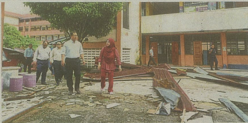
Zahri (front left) visiting SK Petaling Jaya which suffered storm damage to its roof and infrastructure.
