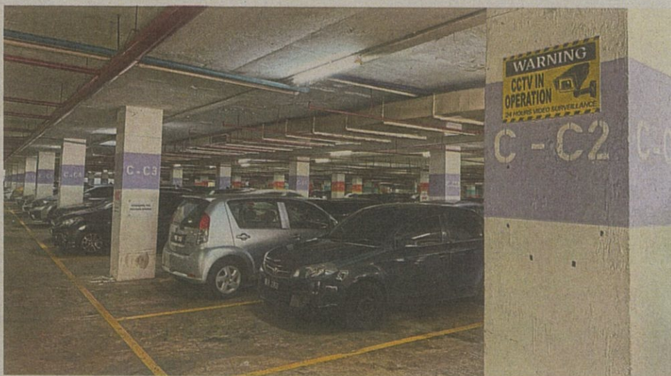
Placing CCTV cameras inside indoor carpark may help to deter criminal activity. — Photos: LOW BOON TAT, FARID WAHAB/The Star
