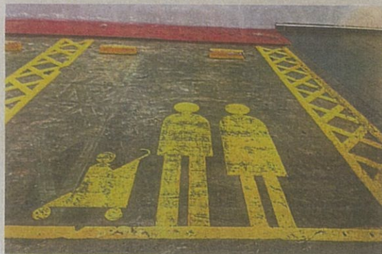
This bay reserved for parents with children is equipped with parking chocks to prevent collision.
