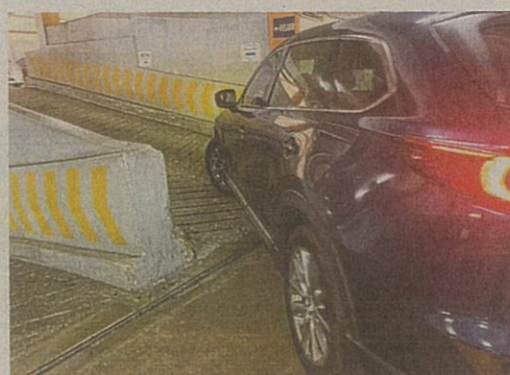
Motorists risk getting their cars damaged by narrow ramps.
